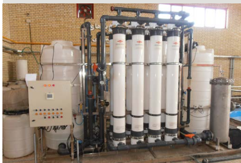
Ultrafiltration Plant in the Morcheh Khort WWTP.
