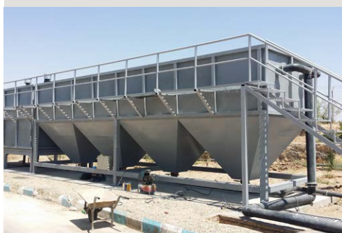
Chemical Sedimentation - Morcheh Khort Wastewater Reuse Plant.
